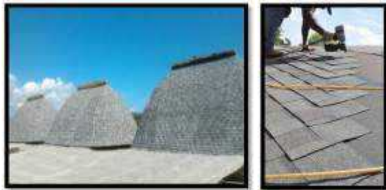
Gambar 136. Atap bitumen (sumber: google image)
