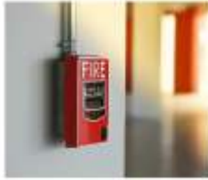
Gambar 85. Jenis Fire Alarm Sumber : http://www.tedsystems.com , 2020
