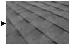
Atap bitumen (material aspal)
