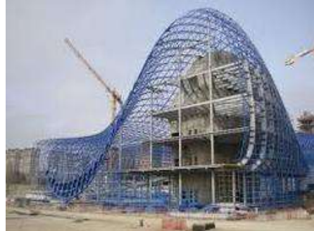
Gambar 4.27 struktur space frame ( sumber : https://www.arsitur.com )
