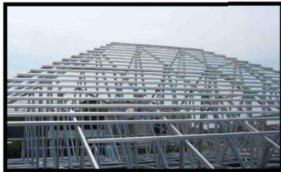
Gambar 5.21 Rangka Atapbajawf (sumber gambar: Gogglesearching/datedownload, 2018)
